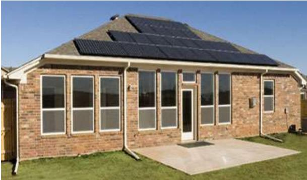
Photovoltaics are placed on the roof of this house and they capture energy from the sun to help offset consumption. This modest home produces as much energy as it consumes in a year, leading to a net zero energy consumption.
